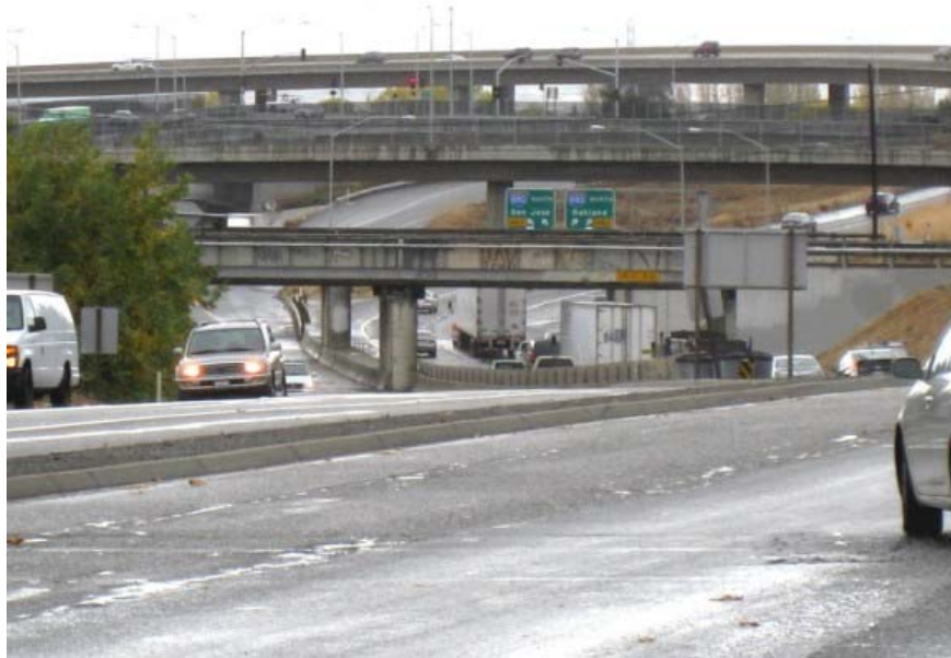
Segment A—looking west from the Warm Springs Blvd. intersection
