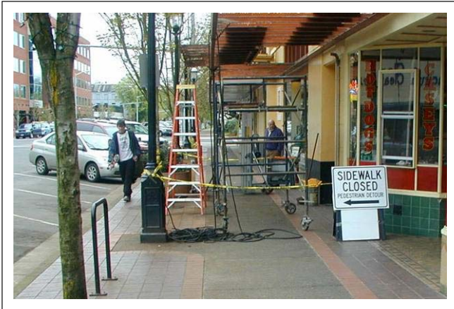
Never block pedestrian access during construction without providing an alternative path
