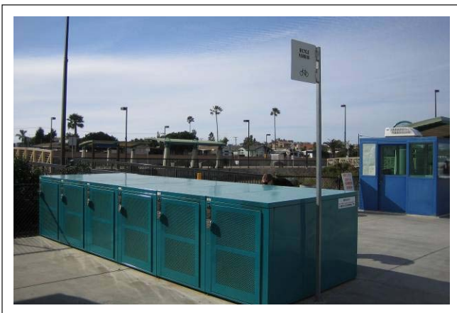
Bike lockers at transit stations should be located to avoid interference with pedestrian activity
