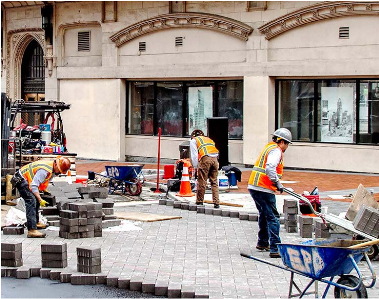
Roadway paver installation at Latham Square.
